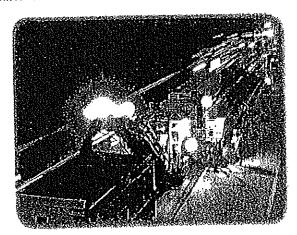
The asphalt placed on this project consisted of SP 19.0, SP 12.5, SP 9.5, and FC-5 friction. The plans included placing ditch pavement at two locations along the project. PBS&J inspector's oversaw the removal of existing bridge guardrail transition and constructed three-beam transition in various locations. They also consisted of removing existing end anchorages and constructing SRT-350 at various locations throughout the project.
